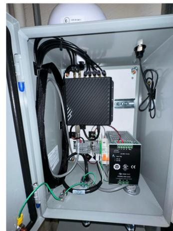
*Cellular modems provide remote site connectivity for ESA and Vibration to the cloud instance of InsightCM™*
