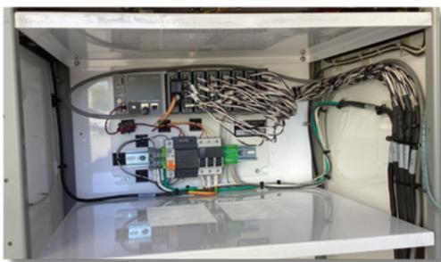
*ESA hardware install in or near Motor Control Center provides high speed three-phase voltage and current monitoring to access pump motor health*
