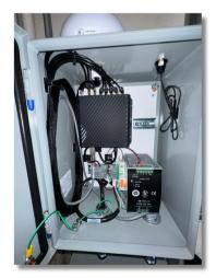
Cellular modems provide remote site connectivity for ESA and Vibration to the cloud instance of InsightCM™
