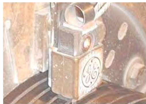
Figure 12: Example of Brush Binding
