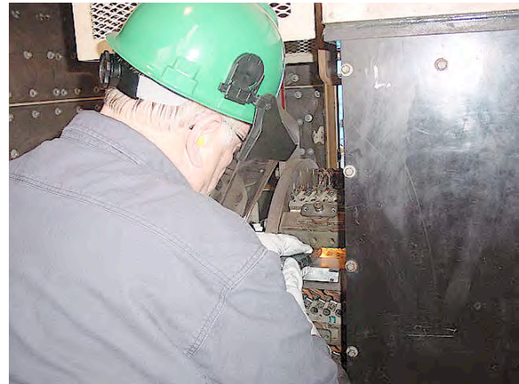
Figure 22 Truing GE 900 MW Rings
